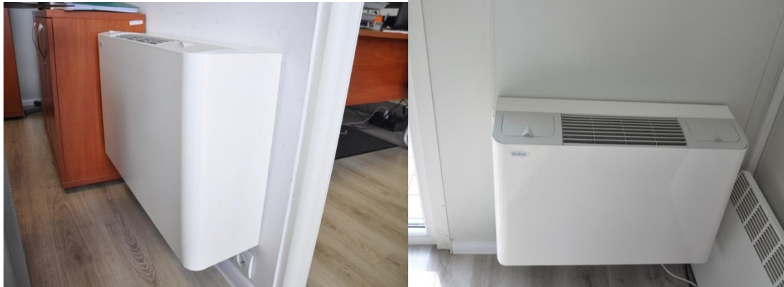
Figure 6-8. Central heating installation (fan coil unit)
