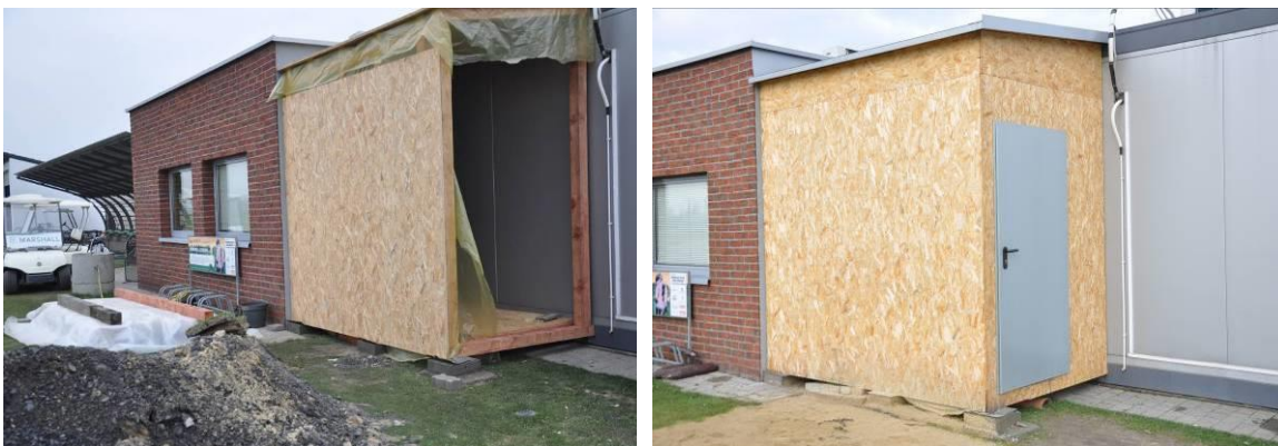
Figure 6-3. Construction of the container
