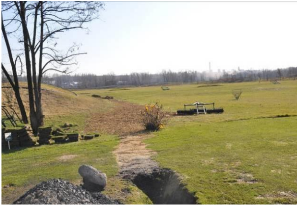
Figure 6-5. Excavation for a pipeline (connection between buffer tank and container)
