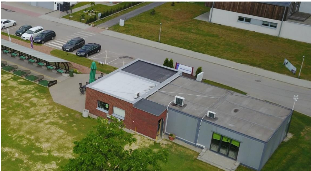
Figure 6-7. Final look over installation container
