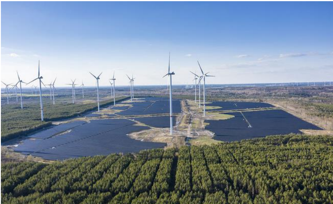
Figure 5-1. (Photo Credit) © TrinaSolar
