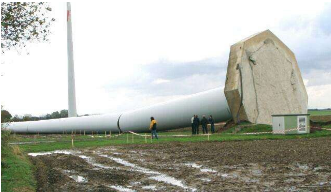
Figure 4-2. Fallen wind turbine facility (windpark-vechigen, 2023)
