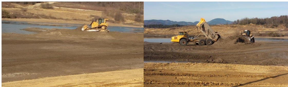
Figure 3-6 Filling the subsidence area in Velenje using Stabilizat
