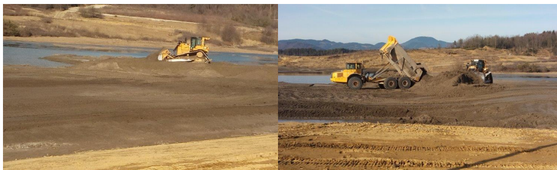
Figure 2-6 Filling the subsidence area in Velenje using Stabilizat
